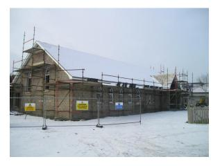
Almost all the slates are laid on the roof of the CPRC church building. All the windows have been fitted and many of the interior door frames. Plasterers, plumbers, joiners, and electricians have made progress, despite the holidays and the very severe weather (for Northern Ireland). I've included a couple of photos: one of the outside of the building and one of the auditorium or sanctuary, which will hold some 128 people.
