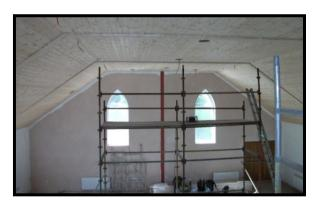
been fitted. Painting is on-going. Some of the next jobs include hanging the inside doors, fitting the kitchen and the "porcelain" in the bathrooms, installing the lift, and varnishing the ceiling in the main auditorium.
